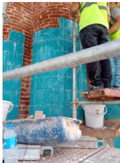
Figure 21, The tiles are applied on the bricks (Resource: Personal Archive)
