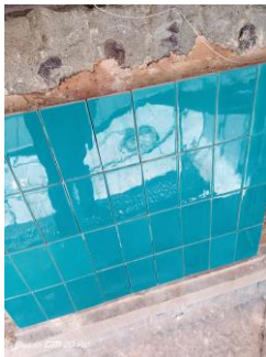
Figure 20, The tiles are applied with khorasan mortar (Resource: Personal Archive)
