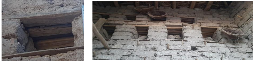
Fig 7. Spaces left for the entry and exit of pigeons
