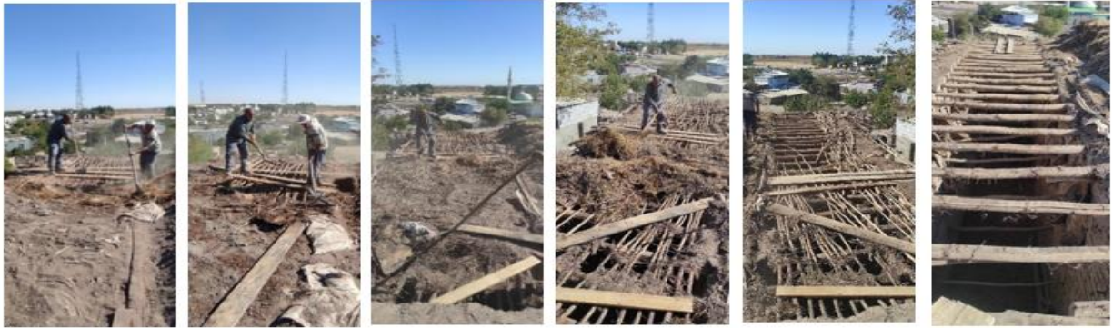
Fig 14. Dismantling of the roof
