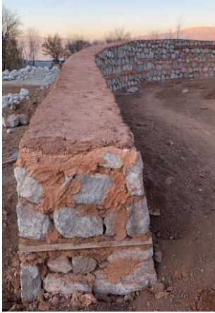
Figure 9. Retaining wall as a wind barrier with horizontal wooden beam inside, December 2019
