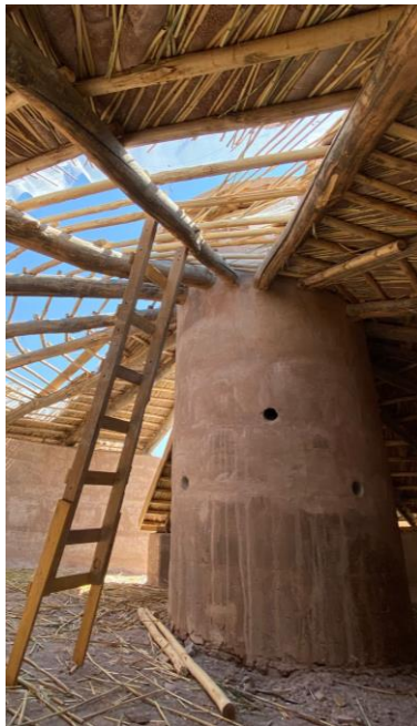
Figure 13. The rammed-earth central column with the openings on the surface, 31 August 2021
