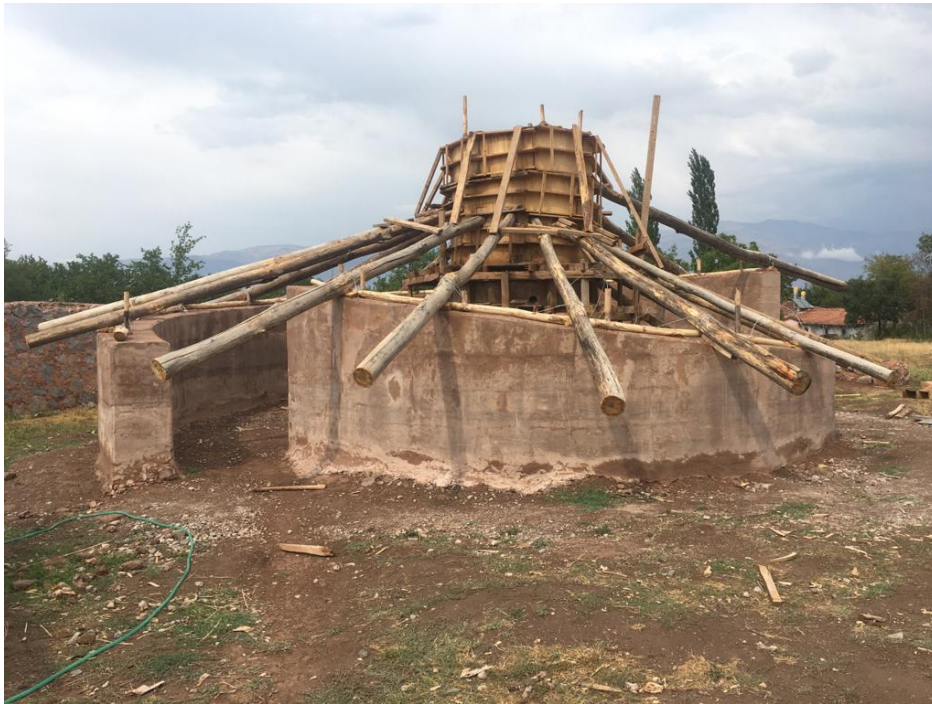
Figure 14. All poplar purlins were carried by the central earth column and attached to certain points on the semi-circle earth walls, 27 June 2021
