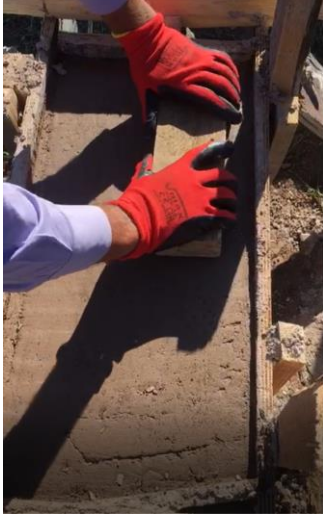
Figure 12. The earth wall mortar was prepared and applied gypsum additive, 30 June 2021
