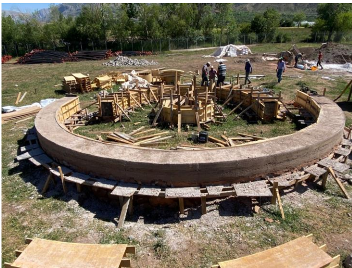
Figure 10. The first 60 cm of the two main earth walls were built., 10 June 2021
