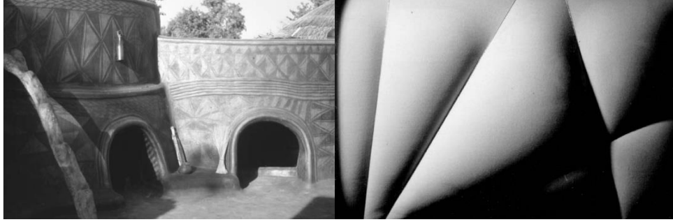
Fig. 5: Houses constructed with wet sculpting technique in Ghana (left), a ceiling design to molded earth which can be constructed pouring mineral loam in formwork of textile stressed by cables (Minke, 2006).
