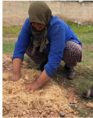
2. The mixture is kneaded by hand for consolidation.
