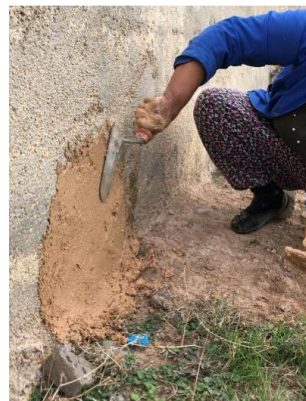
5. The mortar is plastered with a trowel. It is plastered again after half an hour.
